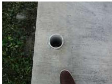
**Open and unused 4" drain pipe at west side flatwork**
