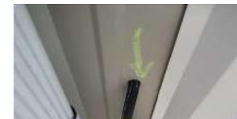
**Seal bond wire cable in west siding**
