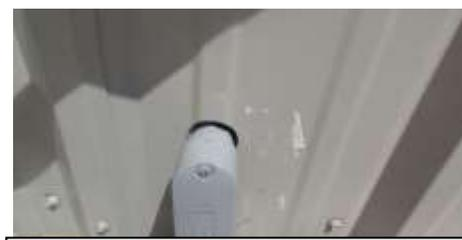
**Seal front electrical LB into wall panel**
