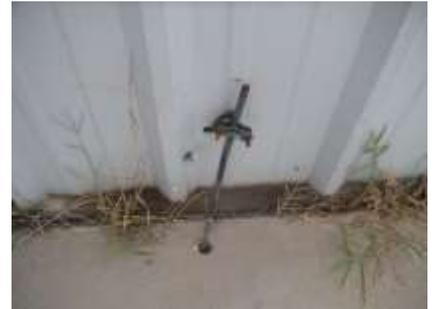
Earth ground not driven flush to grade and old clamp
