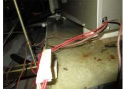
Water in emergency pan and no emergency drain line
