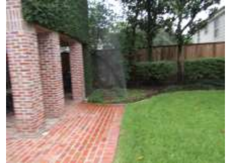
Broken sprinkler head
