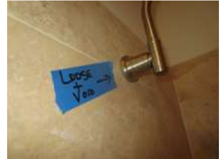
Loose cover with void in second level shower
