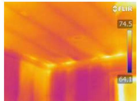
No anomalies on 3 rd level ceiling
