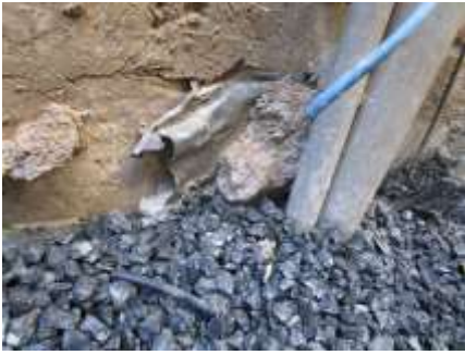
Remove black plastic off west grade beam
