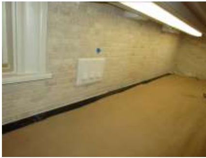
Poor access to disposal switch
