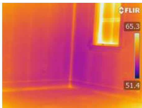
No anomalies in walls of bedroom
