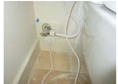
Loose cable for master toilet and seal void
