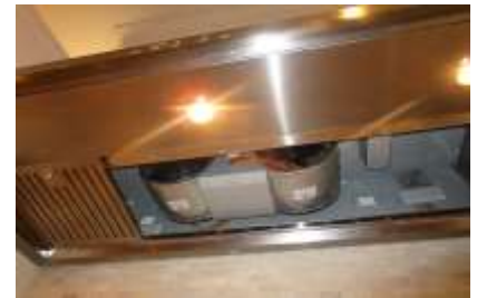
Excess noise off overhead vent in high speed
