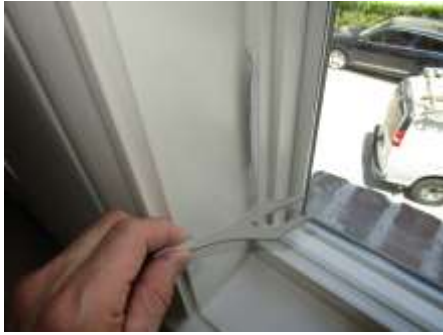
Loose handle for master window
