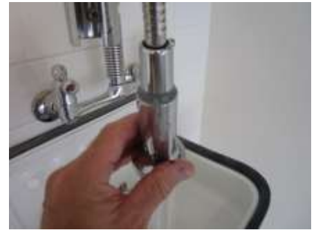
Leak off garage hand-held fixture
