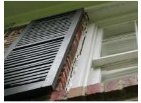
Separation of window and brick
