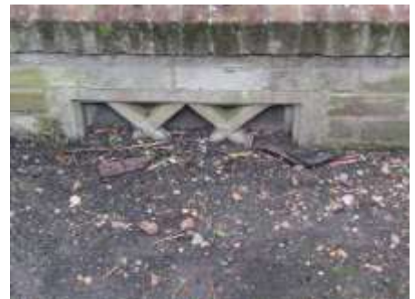
High soils cover half of east vent
