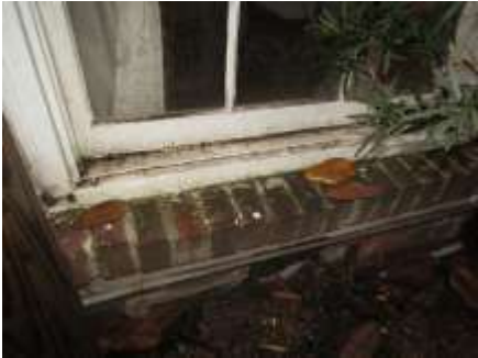
Inverted east windowsill
