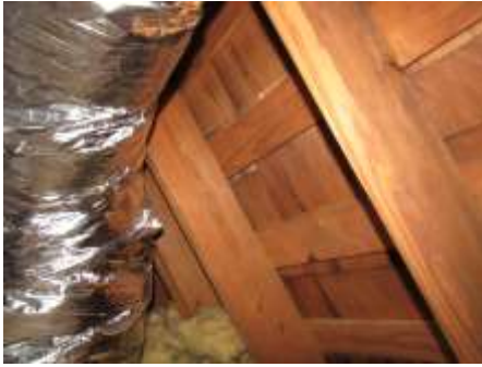
Wood shingles with roof overlay
