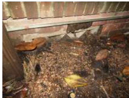
Covered east foundation vent
